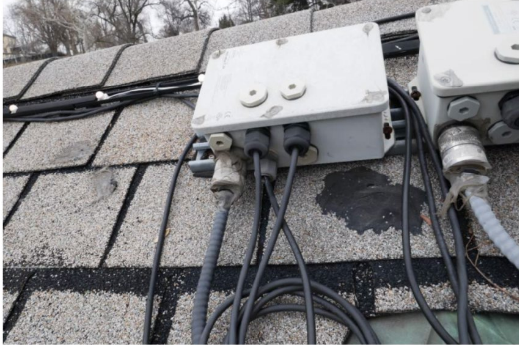
Figure 4. Typical worn power cable condition.
